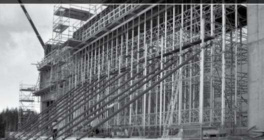
Concrete forming & supporting systems
